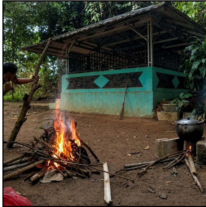
Figure 4. Condition of the Sacred Tomb of Buyut Haer
